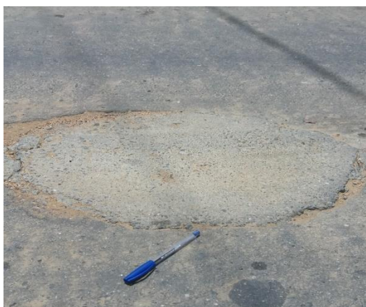
Figura 34 - Remendos (R)
