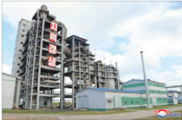
The Kim Chaek Iron and Steel Complex has completed a coke-free production process that features an oxygen blast furnace.
