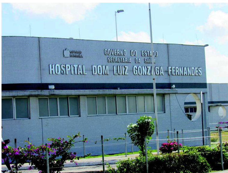
FIGURA 16: Fachada principal do Hospital - 2016
