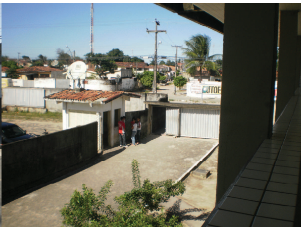
Guarita – Entrada Principal
