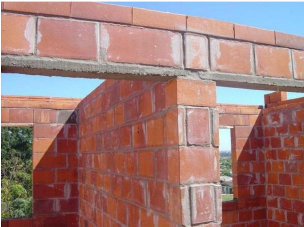
Figura 14 – Verga de concreto moldada in loco
